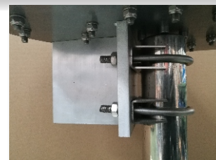
10mm T ALU piece for Mast support
